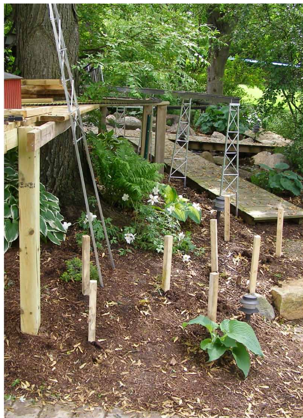
New aluminum support towers completed the tower support between the Willoughby deck and the Avogadro Creek truss bridge. The resulting track support is now stable and strong as well as visually appealing.
