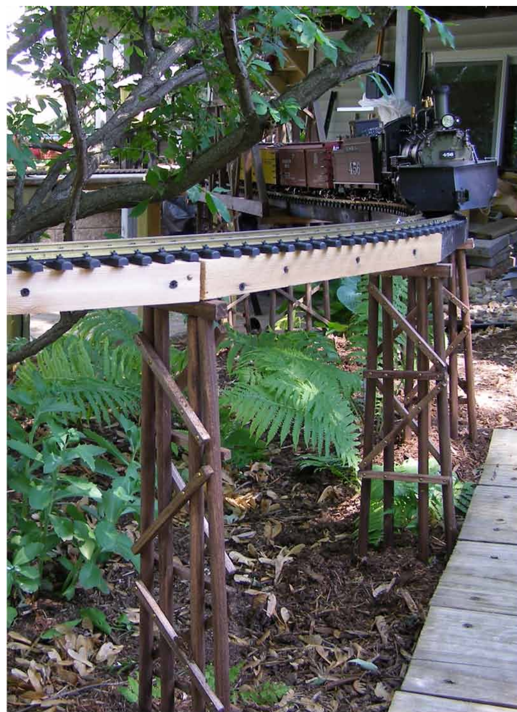
New wooden trestle bents and roadbed deck replaced 2x4 vertical supports and deck planks on the UpperLoop. This improves the appearance as well as making a stronger and stable track support.
